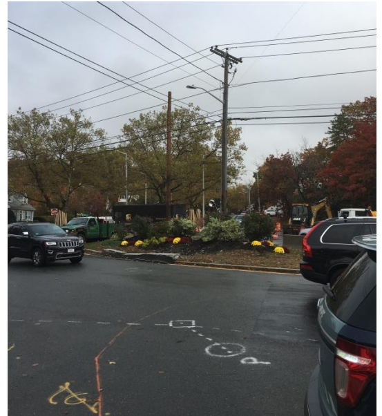
Markings show future locations of conduit and traffic signal poles
